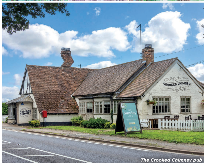
The Crooked Chimney pub
