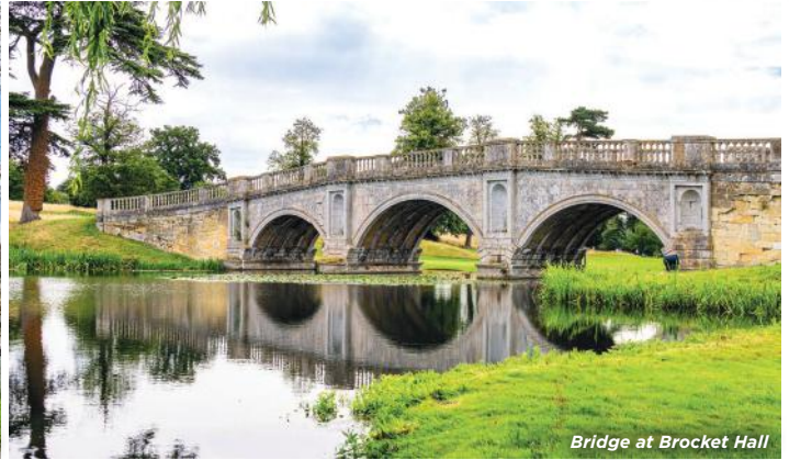
Bridge at Brocket Hall
