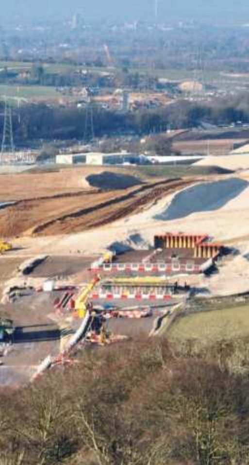
Wendover Dean viaduct site (Photos: Chartridge Photographic)
