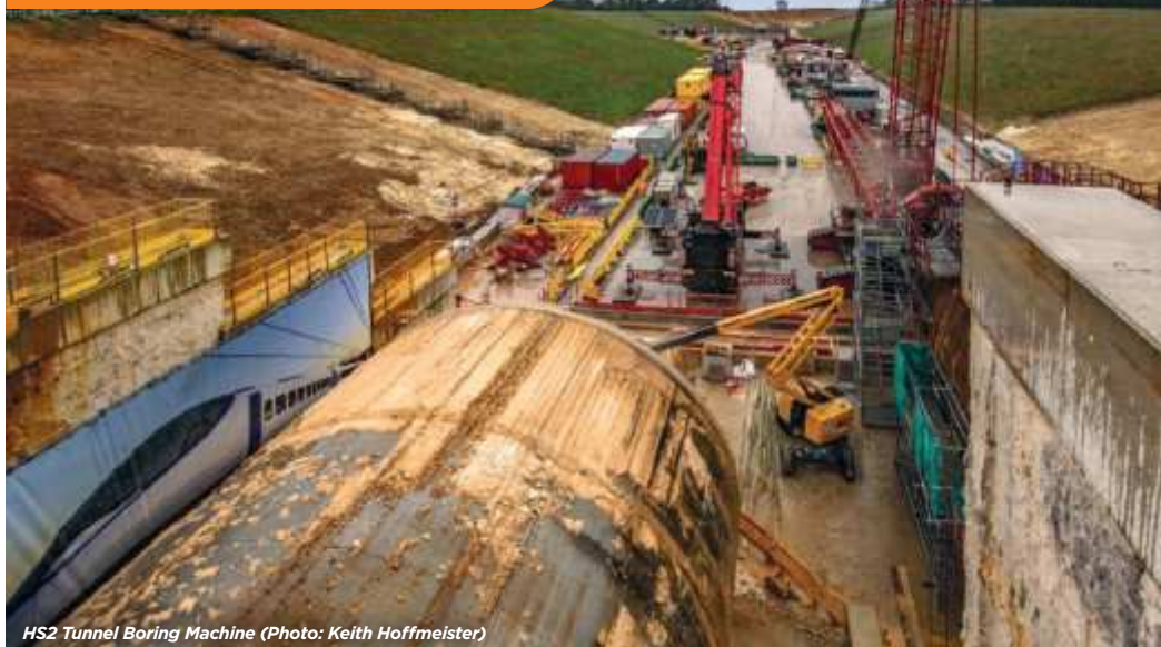
HS2 Tunnel Boring Machine (Photo: Keith Hoffmeister)
