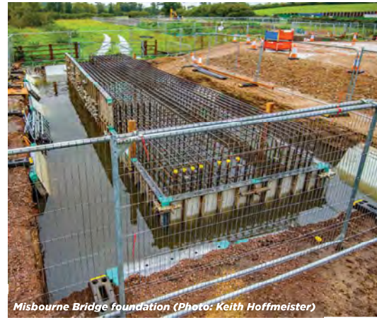
Misbourne Bridge foundation (Photo: Keith Hoffmeister)
