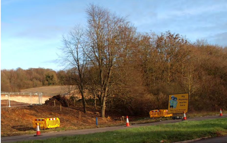
Lane Closure on A413
